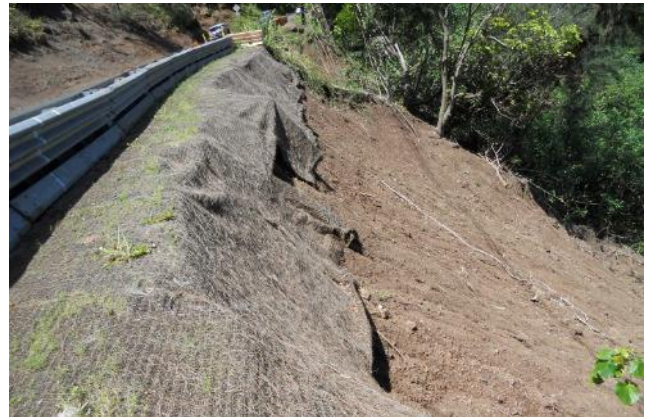
Hillside erosion control prevents road failures caused by heavy rains.
