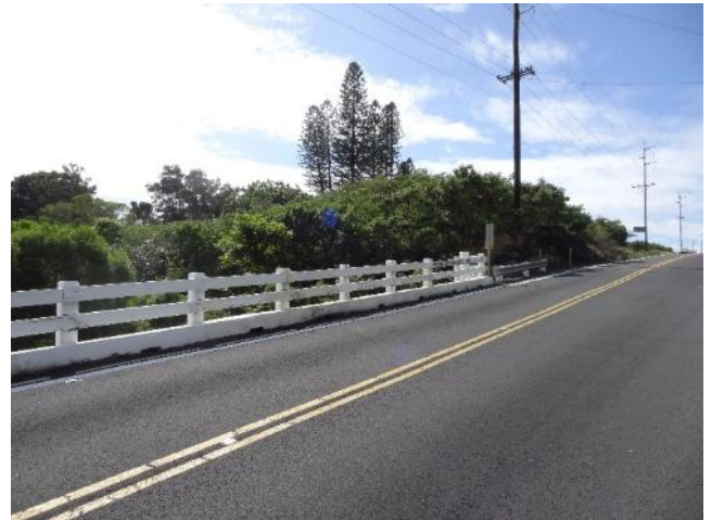
Ninole Bridge, Naalehu, is a crucial link along Mamalaloha Highway, which is the only road around the southeastern side of the island.
